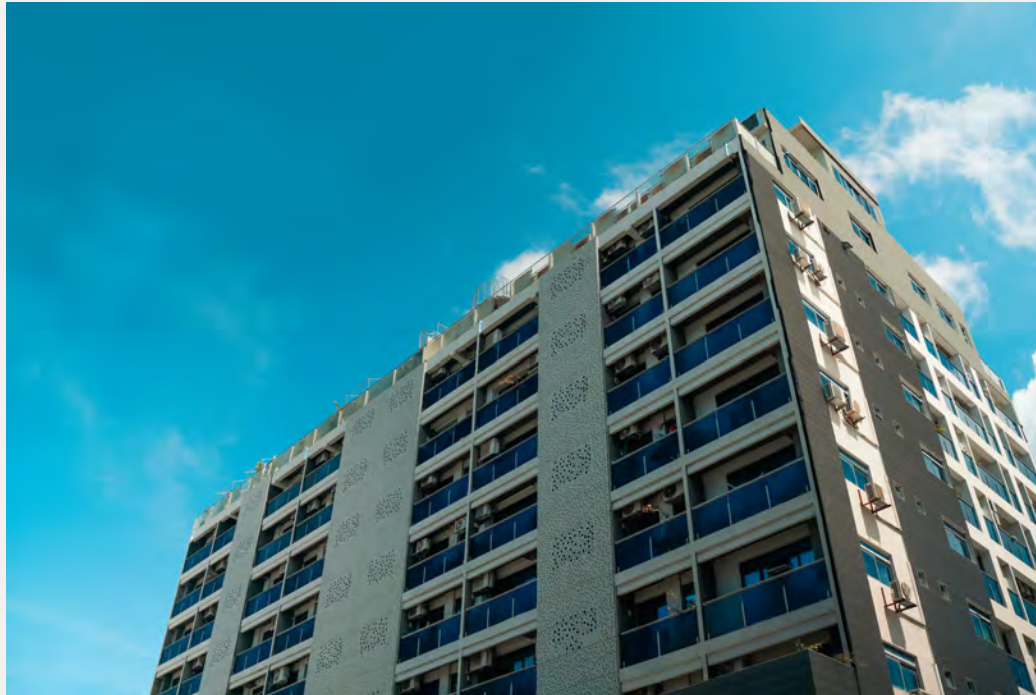
One of our biggest projects in Hulhumale' was the development of a mixed use residential complex, i.e., Marina View – Batch Apartments consisting of 70 Apartment units.
